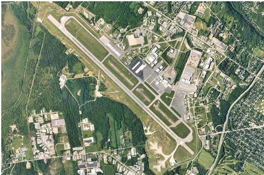
A 2006 aerial photo of the Bangor International Airport. Notice the Christmas Tree alert aprons in the lower right corner of the photo. The Crew Readiness Center can still be seen in the middle of the two Christmas tree aprons.
